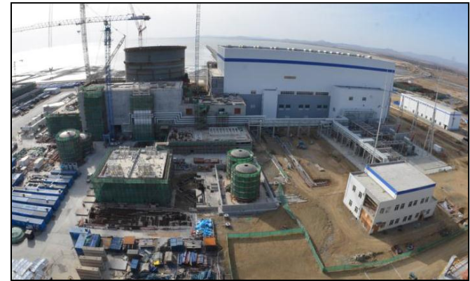
Photos of AP/CAP1000 construction.
